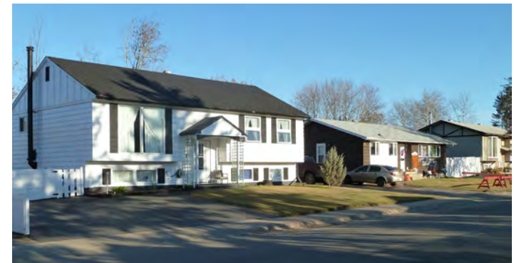
Existing low-density residential
